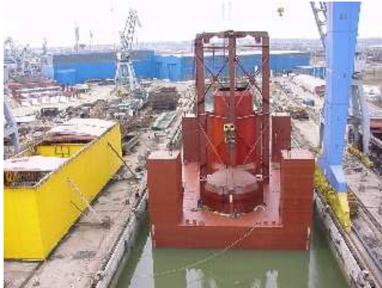
Figure 89 - The AWS 2 MW demonstrator in the building dock at Galati. The domed cap of the floater is resting on the deck of the submersible pontoon prior to fitting of the linear generator
